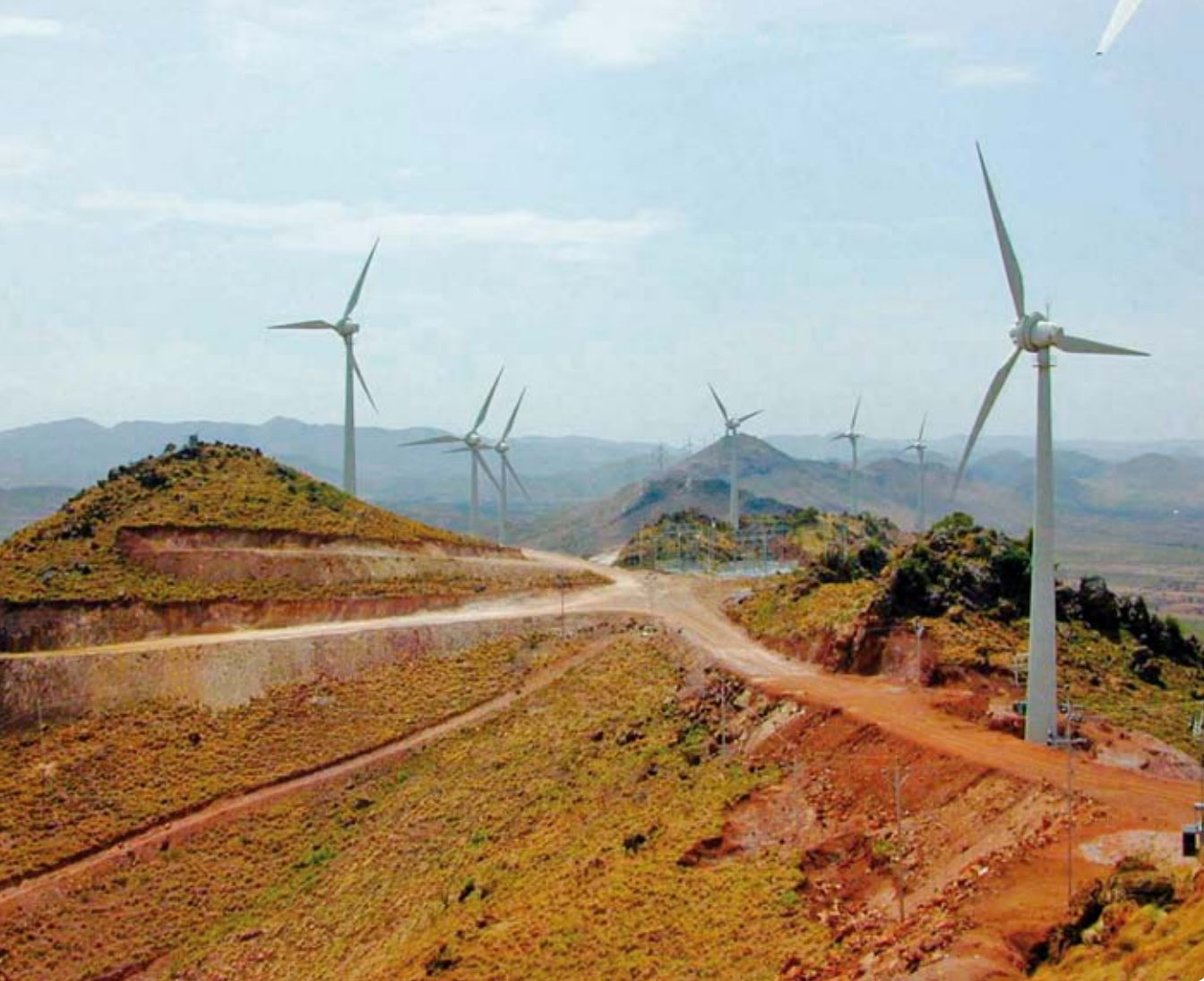
Jogimatti wind farm, Karnataka © Enercon India
