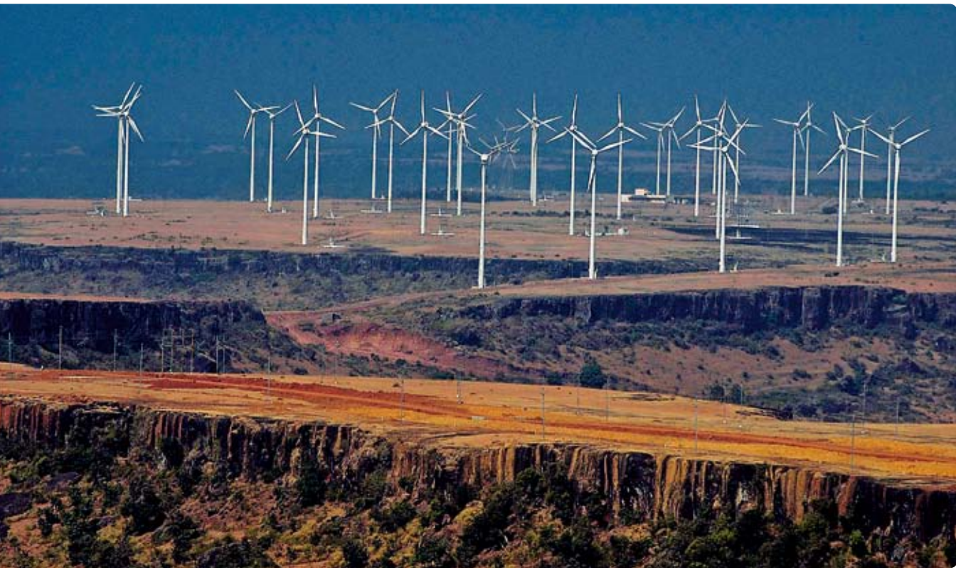
Wind farm in Thoseghar, Maharashtra © Enercon India
