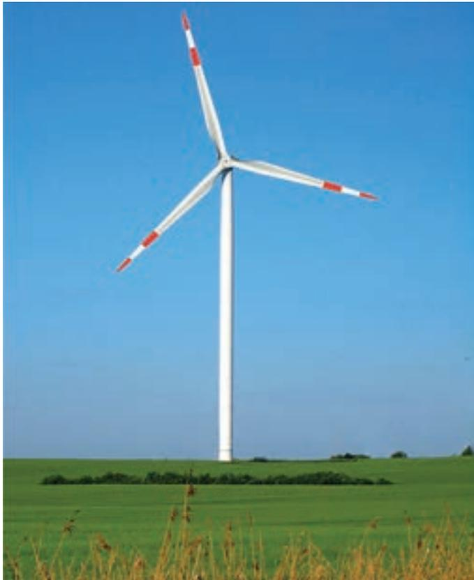
*Figure 5: An example of upwind facing, horizontal axis, 3 blade modern day wind turbine*
