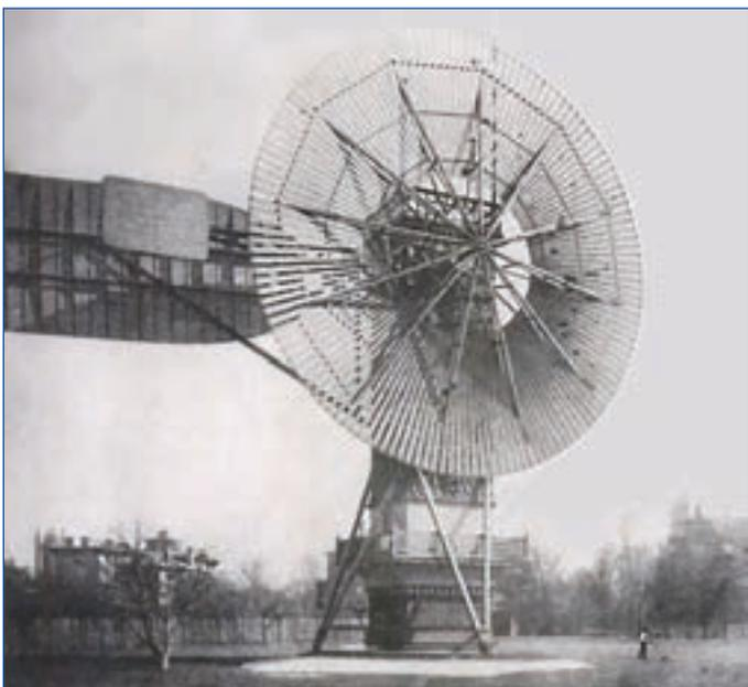
*Figure 4: Horizontal axis design of Charles Brush's windmill in 1888 used for generating electricity (right) (24)*
