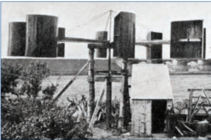
*Figure 3: Vertical axis design of Blyth's windmill*
